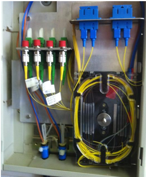
Fig. 10. Experimental FTTH network terminal at Technical University of Košice.
